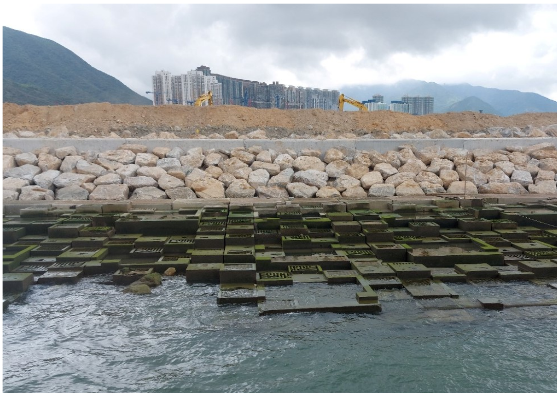
Photo 4 – Natural Rock Material/Planting for Artificial Seawall
